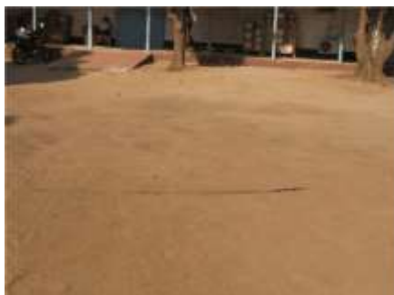
A live electric cable that has come to the surface.
