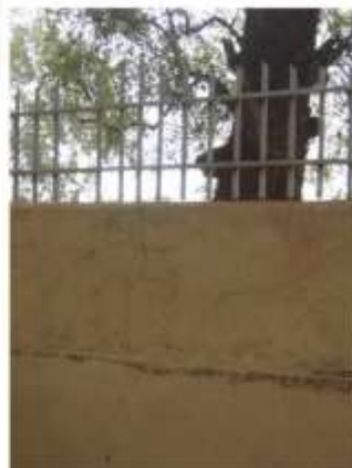
A tree, which is too close to the security wall and wrought iron bars, is compromising both structures.
