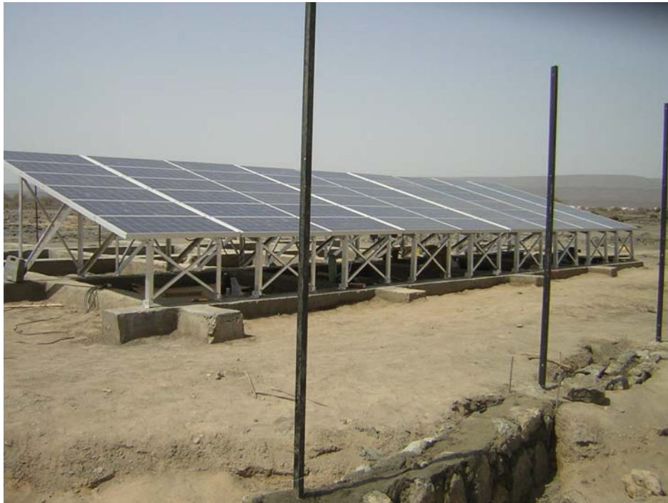
Dorra solar panels provide the pump with energy
